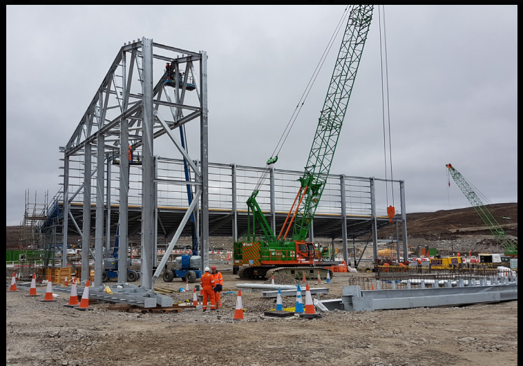
The steel structure at Stronelaig was AJ's largest project to date.
