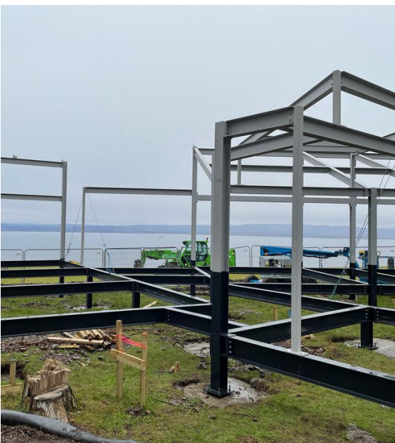
The Westerwoods private house under construction
