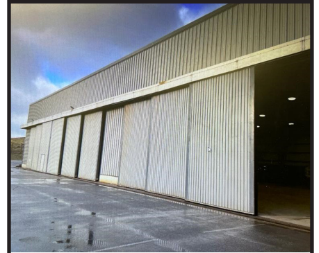
The hangar door at Sumburgh Airport
