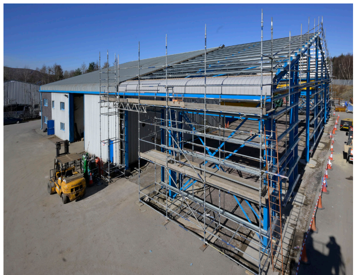
The extension at NEWCo is well underway
